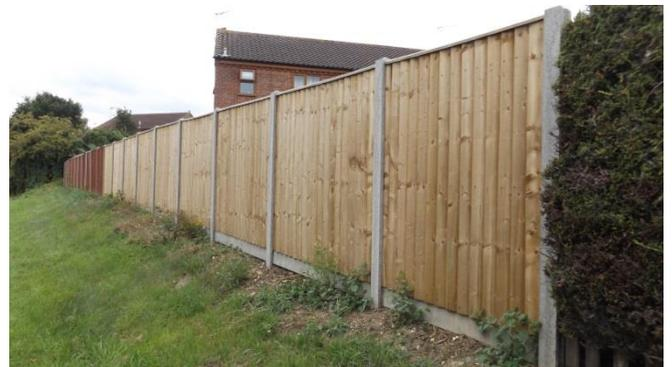
At the side and back we recommend 1.8 m high fences. A good design is a 1500mm fence with 300 mm trellis above which provides a good level of security and makes it difficult to climb.
